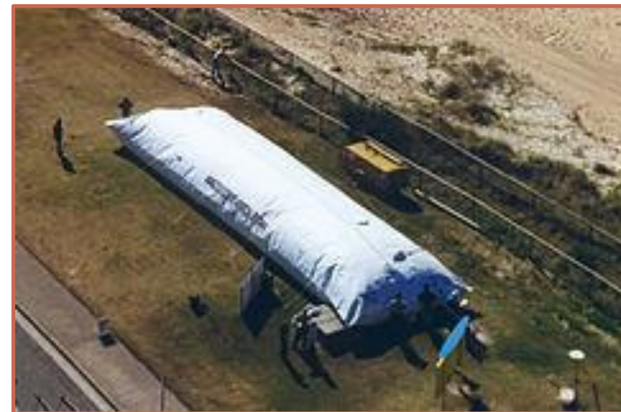
Geotextil sand bag
