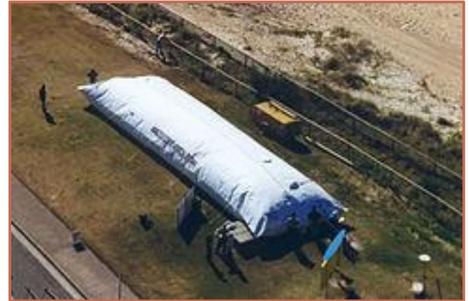
Geotextil sand bag
